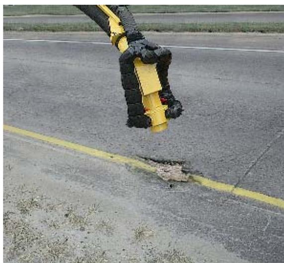
**Figure 3. Hole Being Cleaned for Repair**
