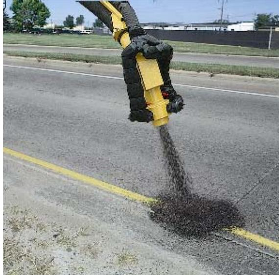
**Figure 4. Aggregate and Asphalt Blend Being Applied**
