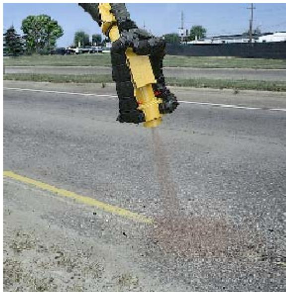
**Figure 5. Coat of Dry Aggregate Being Applied**
